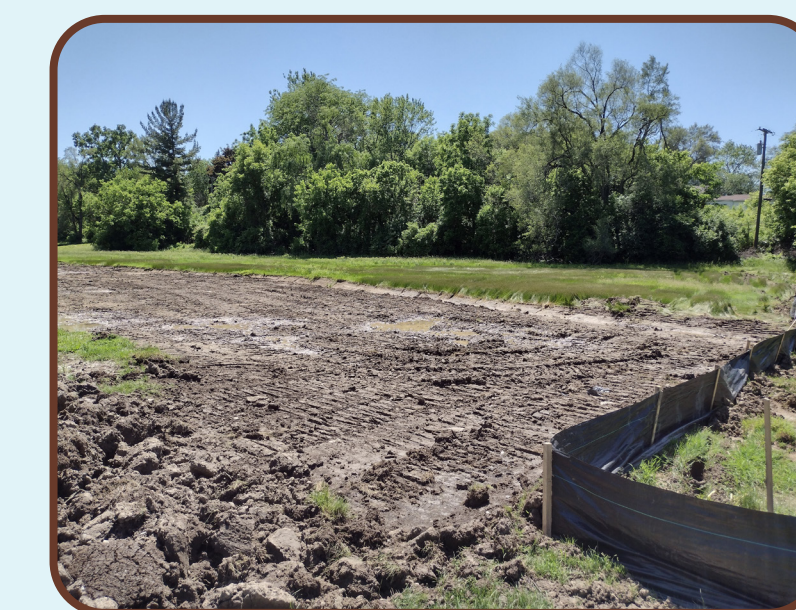
Earthwork to expand existing wetlands to better manage stormwater
