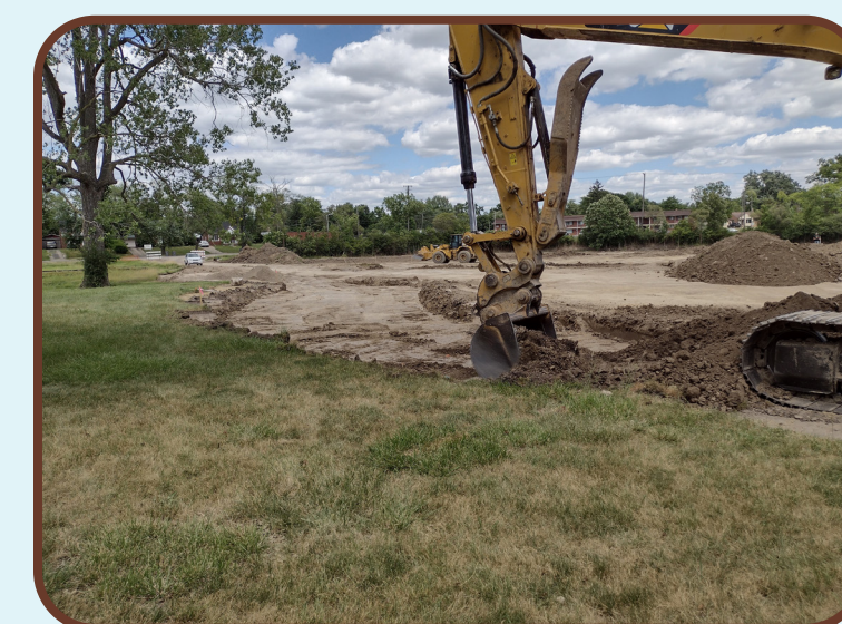
Earthwork to expand existing wetlands
